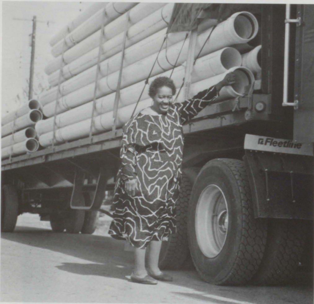
Anticipating better times for the community, Mayor Jones greets the first truck load of pipes to be used to repair and update the town's water distribution system.
