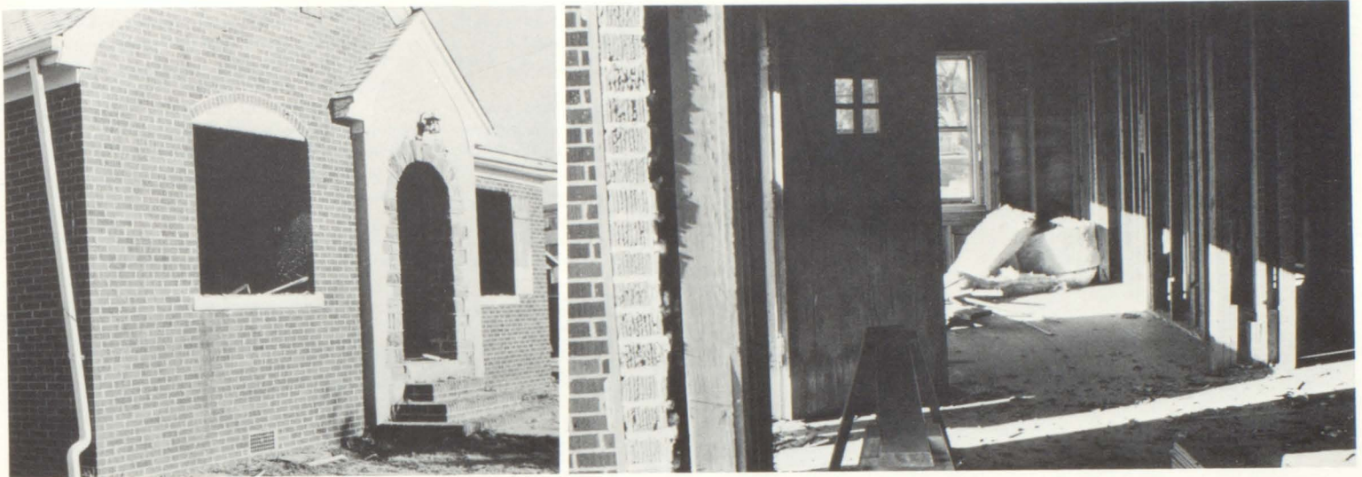
Faculty Cottages are still in the process of being renovated
