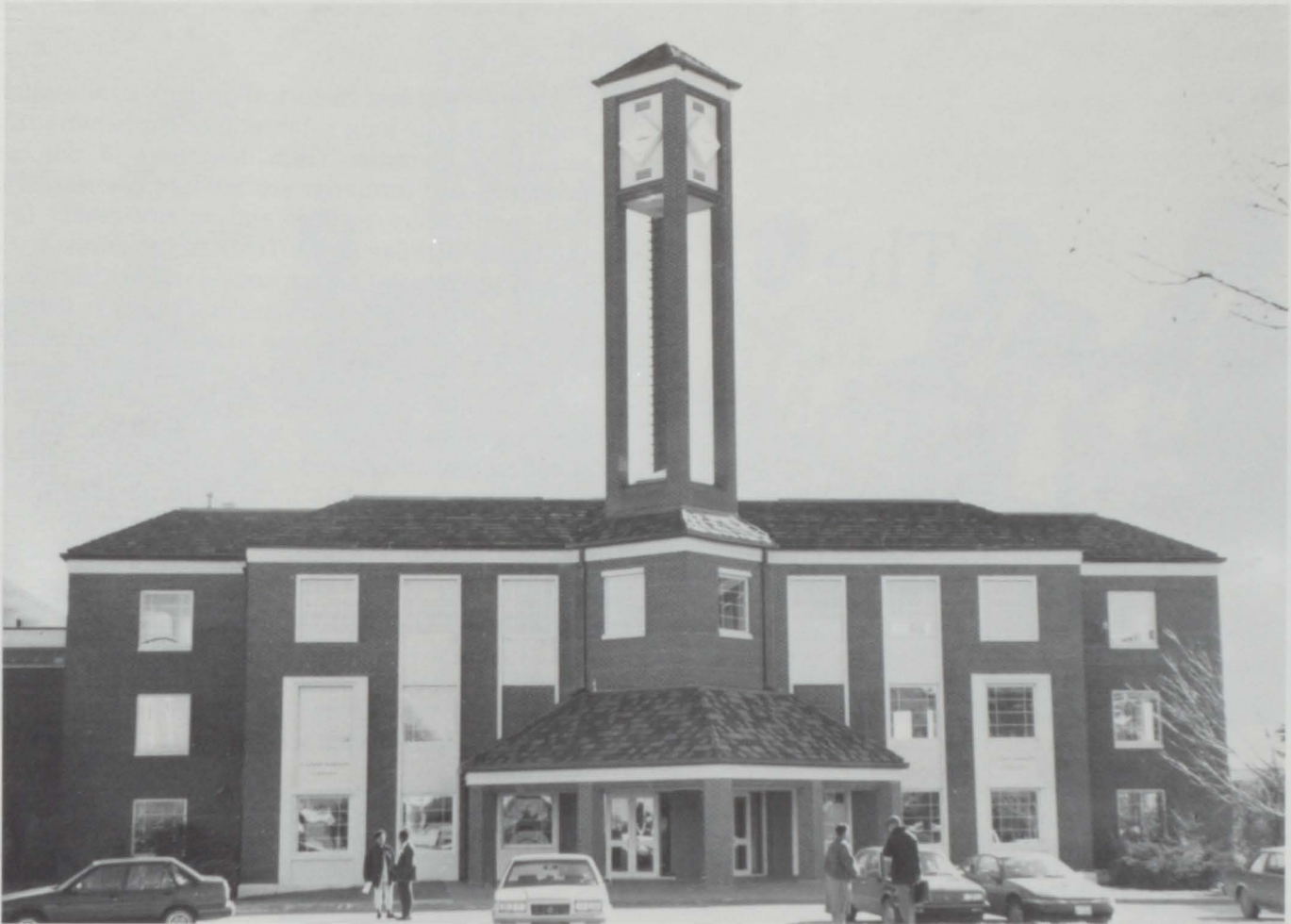
The new bell tower on the G. Lamar Harrison Library points in the direction that Langston University will take in providing quality educational opportunities for the coming century.
