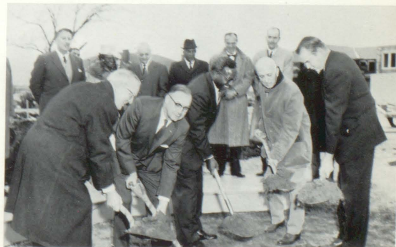
Leading state officials were participants in the Groundbreaking ceremony initiating the now completed two million dollar building project: left to right, Dick Fogarty, R. L. Crowder, President Hale, the late Louis Ritzhaupt, and Governor Bellmon.
